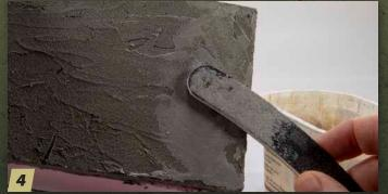
After the mud dried, I wet-sanded the surface with a coarse sanding stick — about 100 grit. I frequently dipped the sanding stick in water to wash away the caking mud.
